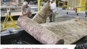
A nylon reinforced vapor barrier keeps out moisture, pests and allergens, and a thick blanket of insulation is the foundation for a comfortable and energy-efficient home.
