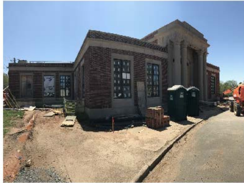
Glass installation on main level
