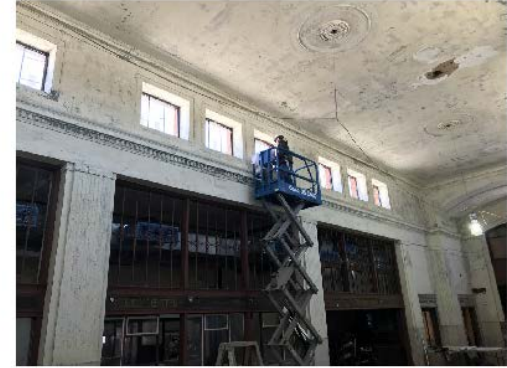
Installing glass in clerestory
