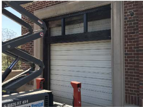
Cast iron storefront at tenant entry
