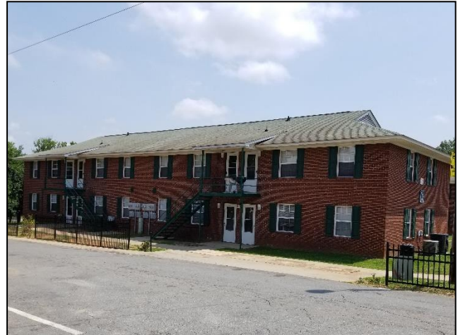
New Hope Manor Rehab
