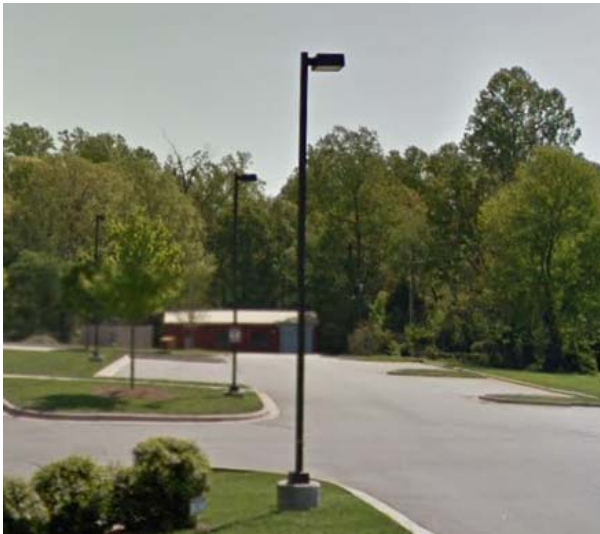
PARKING LIGHTING ON SUBJECT
