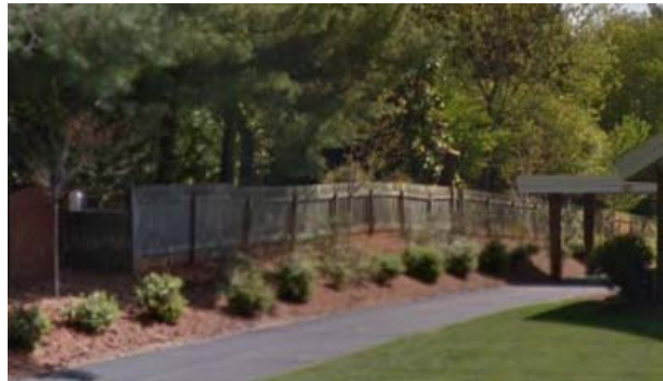
FENCING REAR OF MILLER CROSSING
