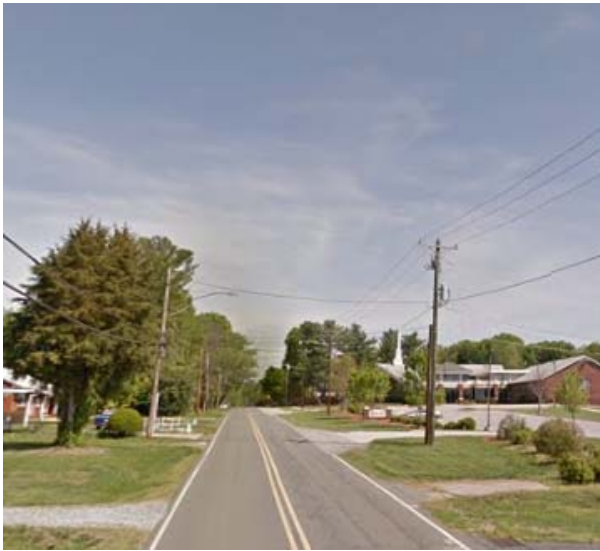
POWER LINES ALONG EBERT STREET
