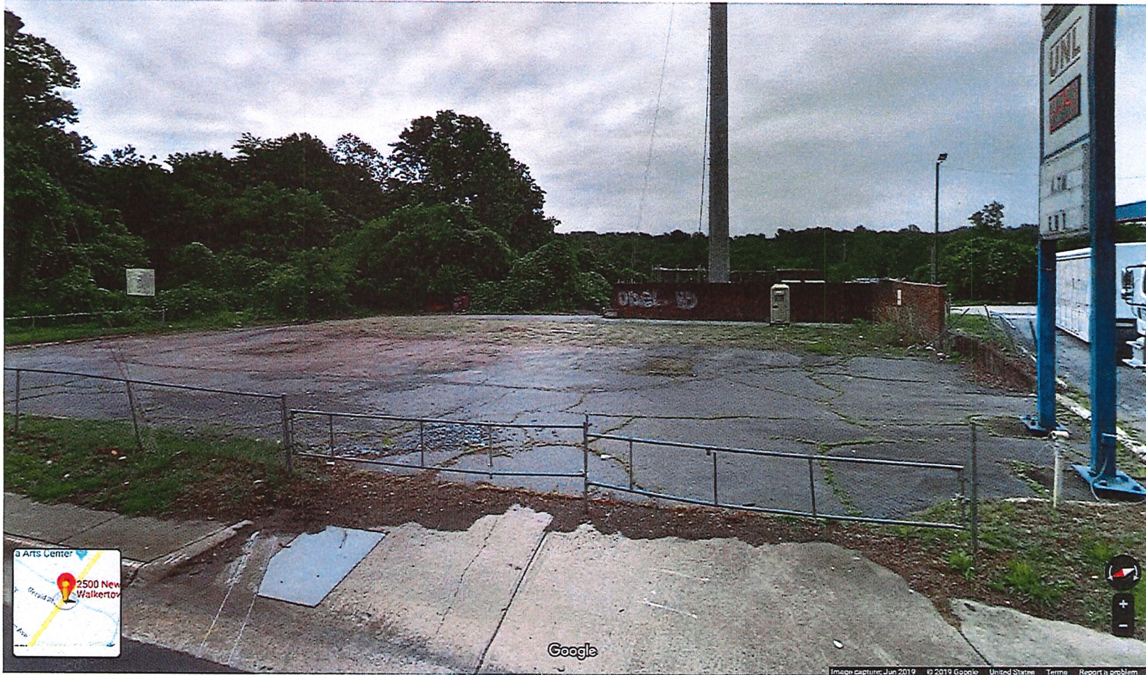
2500 New Walkertown Road Site of New Construction
