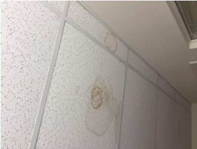
Damaged ceiling tiles from roof leaks
