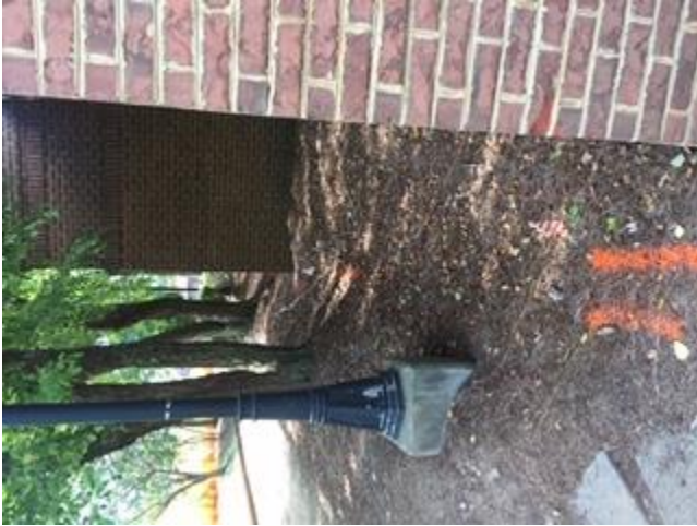
Birch trees in close proximity to build could be potentially problematic to foundation in future.
