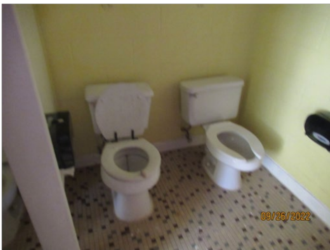
View of the conditions of the plumbing fixtures not ADA compliant.
