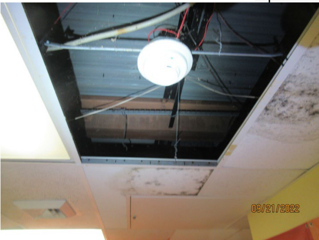
View of interior ceilings - Needs to be replaced due to leaks.
