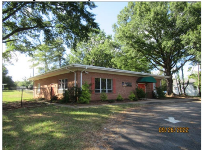
Large oak trees adjacent to the structure are blocking up roof drainage and could damage building foundations. Recommendation is to remove trees.
