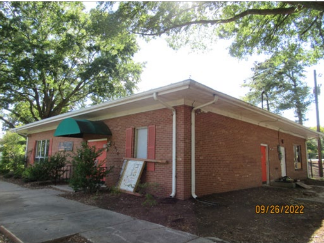
Facade View - Facade needs to be pressure washed / and exterior window are single pane and should be replaced for energy efficiency.
