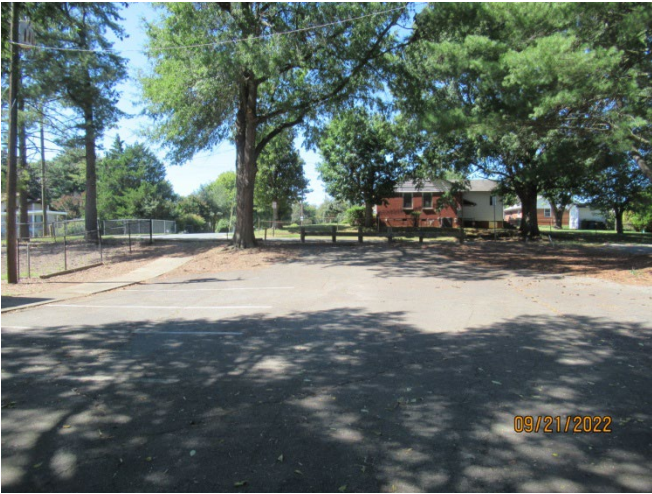
Parking lot: Severely distressed, recommend milling and repaving. Seal coating and patching would buy a few years of use.
