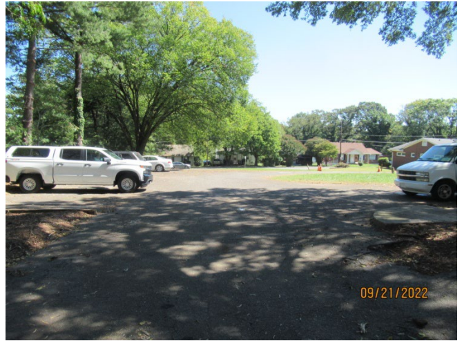
Parking lot: Severely distressed, recommend milling and repaving. Seal coating and patching would buy a few years of use.
