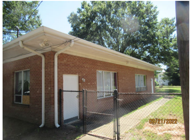
Facade View - Facade needs to be pressure washed / and exterior window are single pane and should be replaced for energy efficiency.
