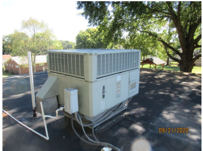
EPDM roof severely deteriorated and need of replacement. Due to the extremely poor roof condition, tear off to the deck is required to verify roof decking is structurally sound.
