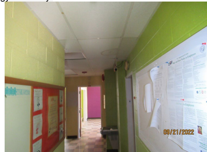
View of interior ceilings - Needs to be replaced due to leaks.
