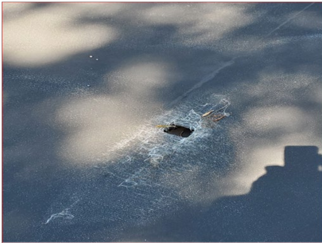
EPDM roof severely deteriorated and need of replacement. Due to the extremely poor roof condition, tear off to the deck is required to verify roof decking is structurally sound.
