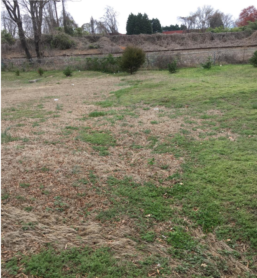
View looking east along the drainage path back toward the railroad property.
