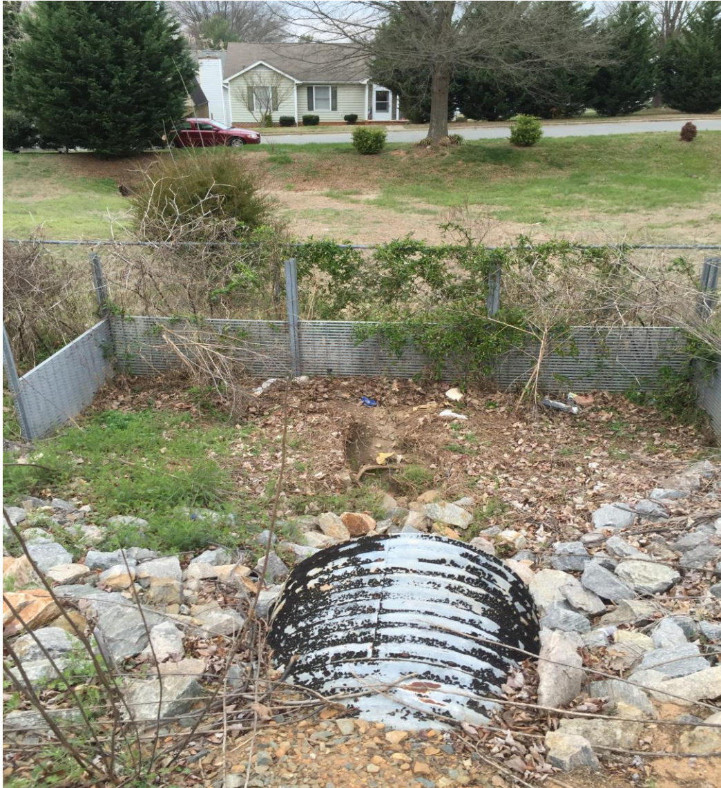
View looking west from rail road into Ms. Pollock's property.
