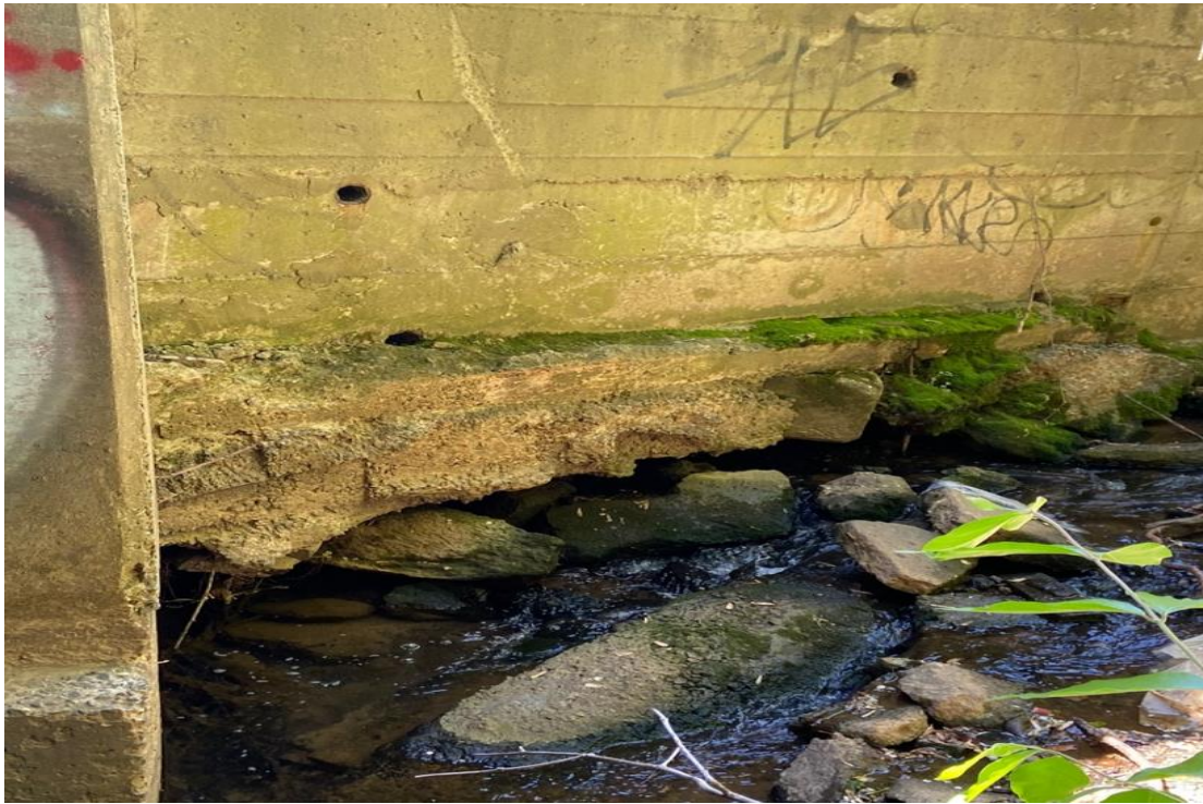
Undermined headwall
