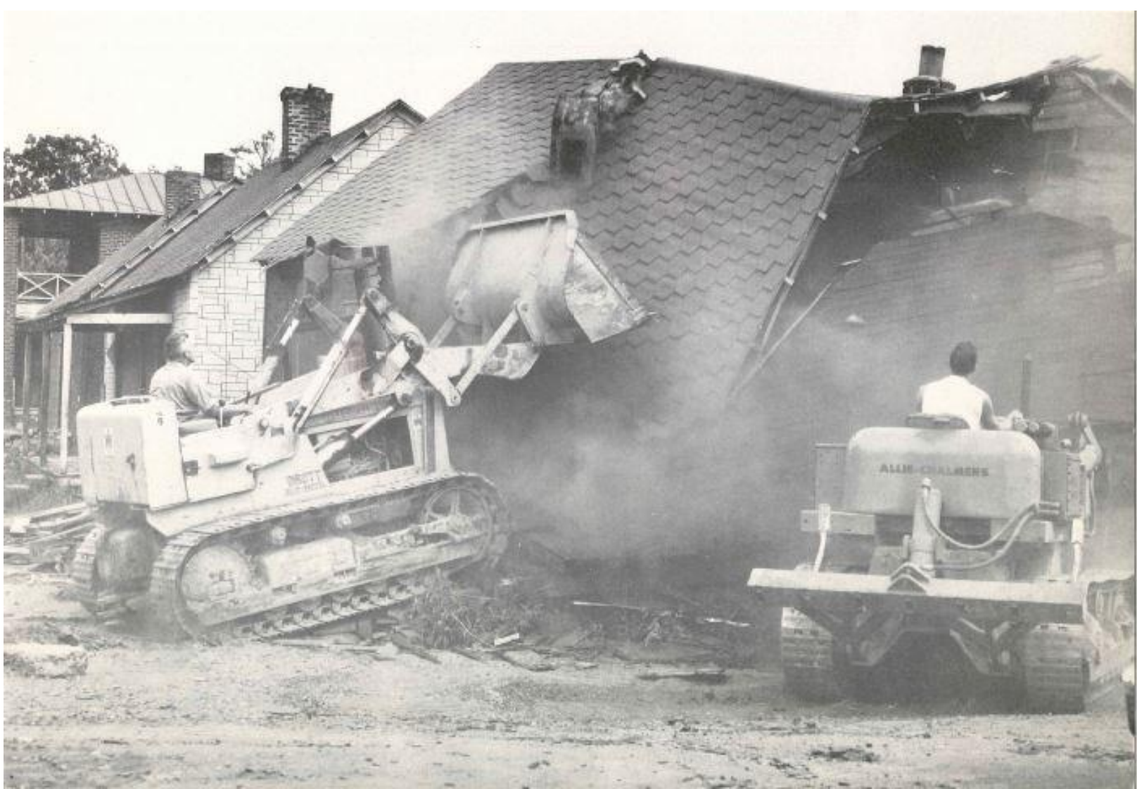
First demolitions in GNRP Project 1 at Eleventh and Ridge Streets, September 13, 1961
