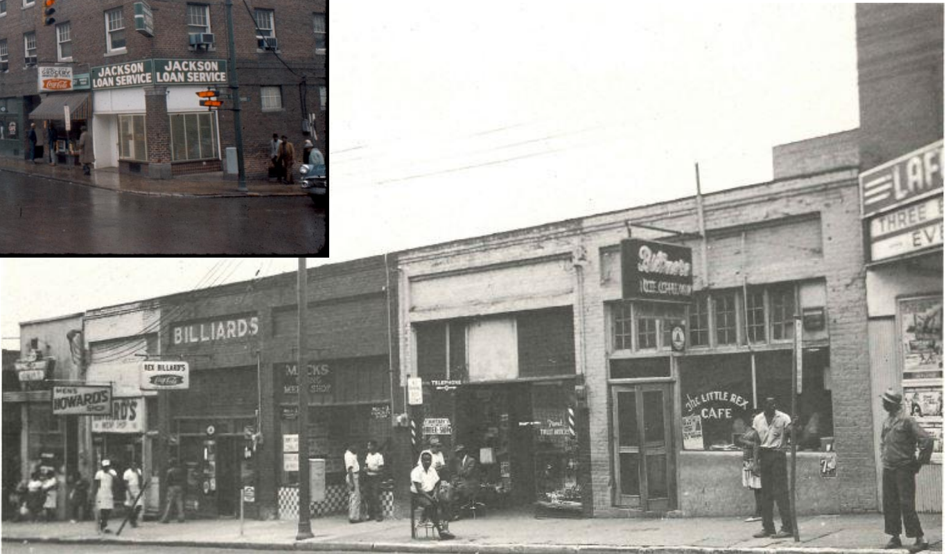
Church Street before renewal, left Fourth Street before renewal, right
