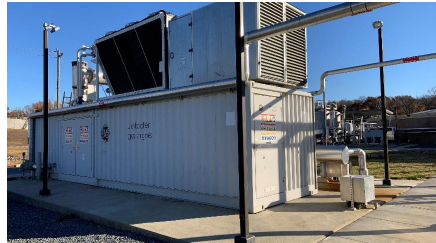
Muddy Creek Wastewater Treatment Plant biogas generator
