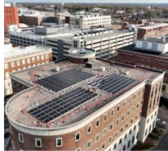
70 KW Solar PV system on Bryce A. Stuart Building
