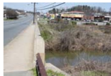
A separate pedestrian bridge could replace this sidewalk along the Peters Creek Parkway bridge over Salem Creek.
