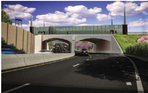
This artist's rendering shows the clear noise wall to be installed along the bridge that will carry Peters Creek Parkway over Business 40 after it is rebuilt.
