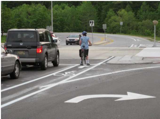
Example of a Class II dedicated bike lane
