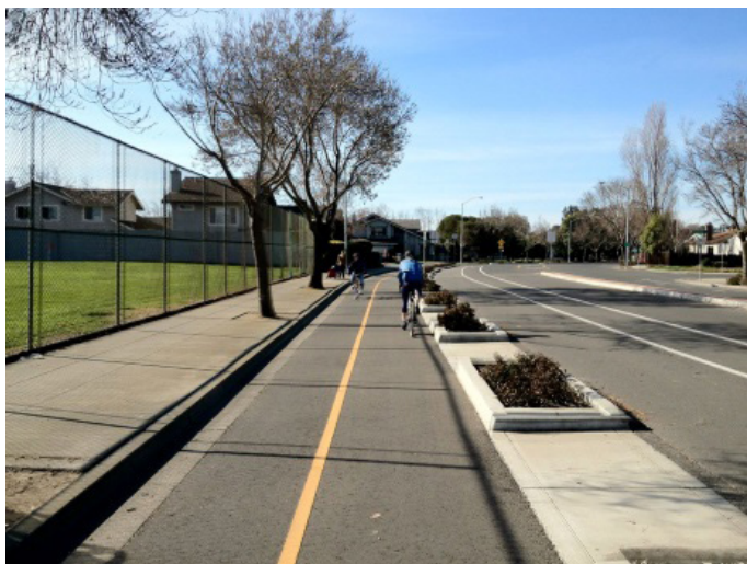
Example of a Class IV protected cycle track
