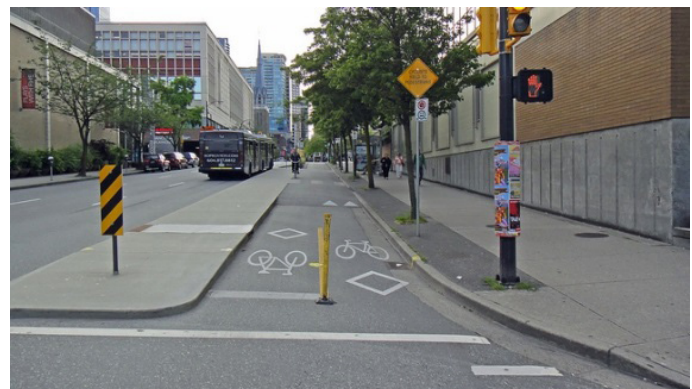
Example of a Class IV protected cycle track
