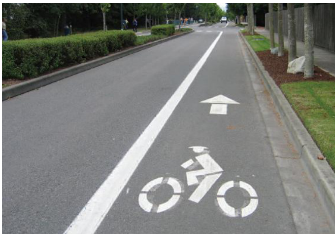
Example of a Class II dedicated bike lane
