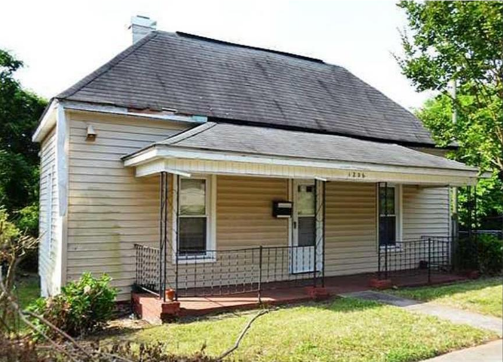
1206 Excelsior St – 2 Bedroom, 1 Bathroom (950 sqft)
