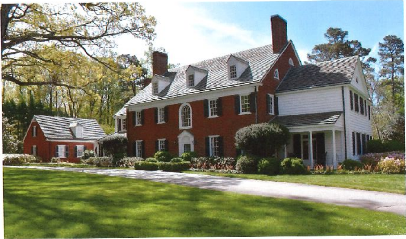
Façade (north elevation), northwest oblique
