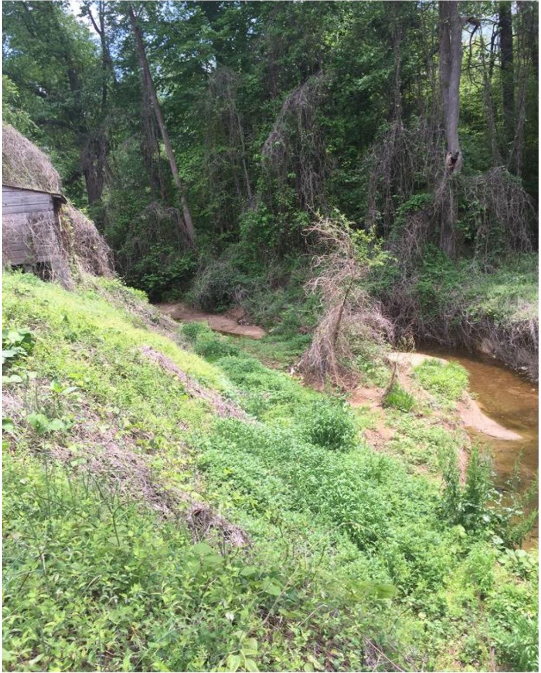
View looking southeast (upstream) behind properties on Cassell.
