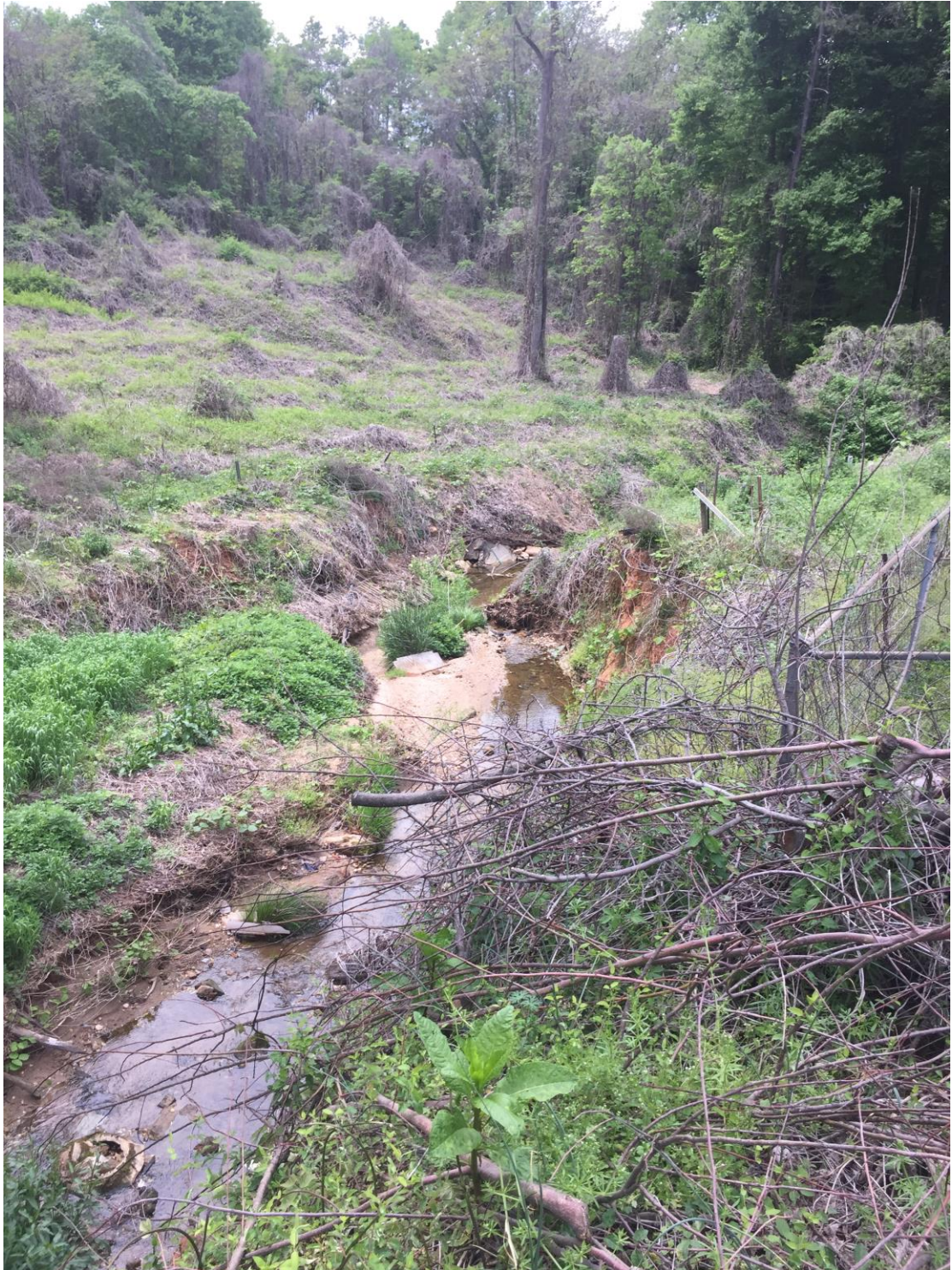
View looking northwest (downstream) behind properties on Cassell.
