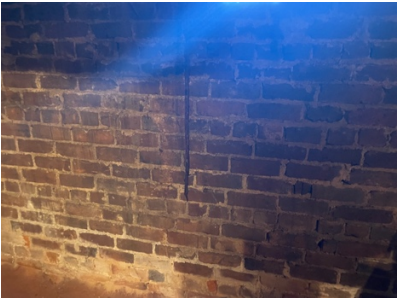
Brick foundation, south cellar, west wall, visible from interior
