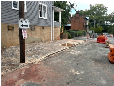
Foundation, prior to rehab
