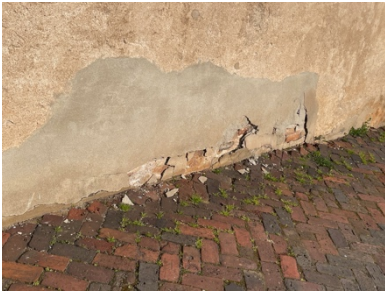
Foundation, prior to rehab
