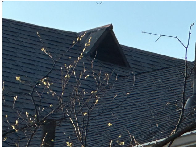
Roof vent illustrating east to west position of 1840 gable
