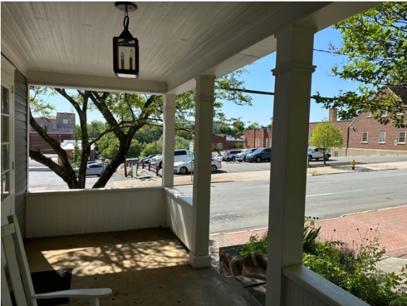
North porch, facing street
