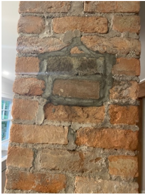
Internal chimney, north
