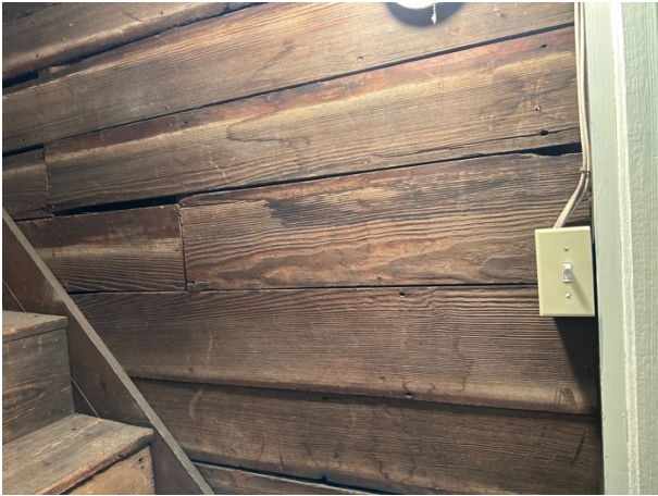
Original attic staircase
