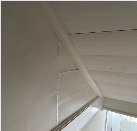
1800s floorboards used to cover entrance to second-floor southwest bedroom during 1920 duplexing
