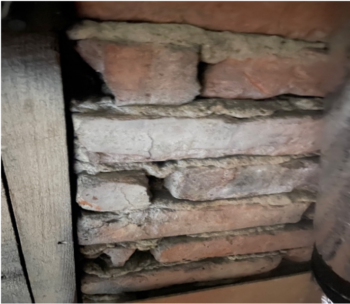
Brick Nog, south cellar
