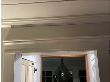
Doorway, south side, first floor
