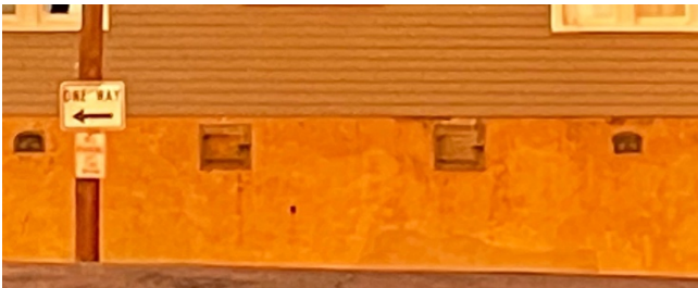
Coal grates feeding north and south duplex furnaces
