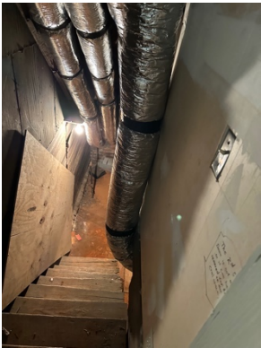
Stairway to cellar, north
