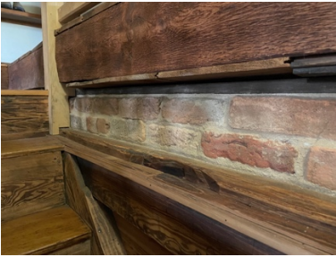
Top of attic stairs
