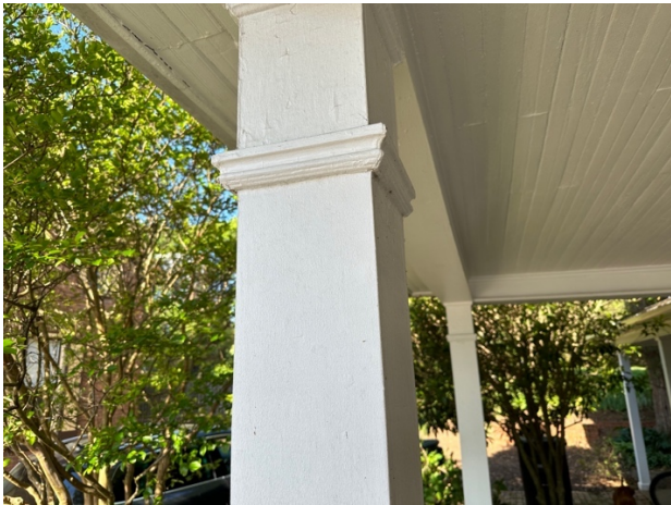
North porch pier with decorative molding
