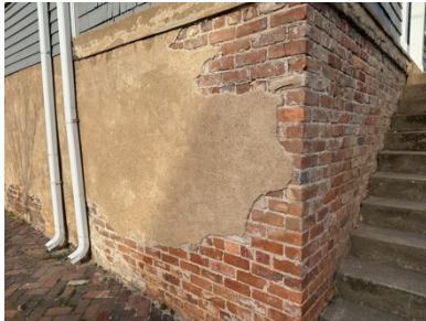
Foundation, after rehab
