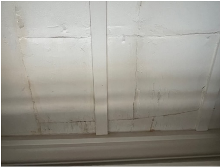
Pull-down hatch, south
