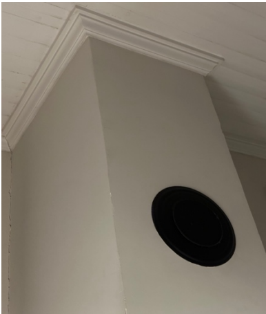
Stovepipe cover for 1920 interior chimney
