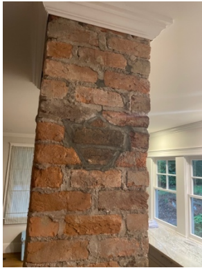
Internal chimney, south
