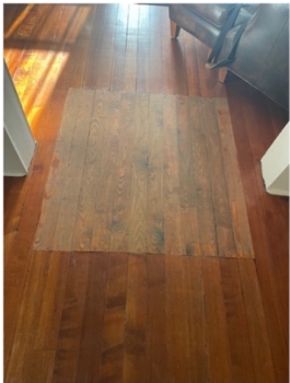
Cutout over coal furnace, south
