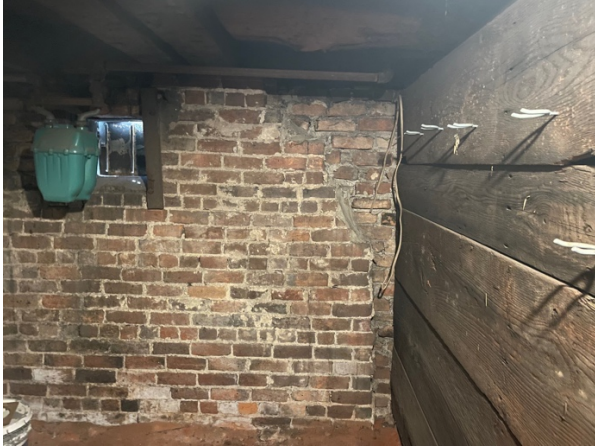
Floorboards from 1800s Repurposed in 1920 Dividing Wall
