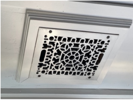
Decorative grate over duct, north
