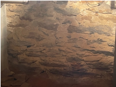
Stone foundation, south cellar, south wall, visible from interior
