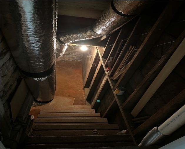
South side cellar stairs
