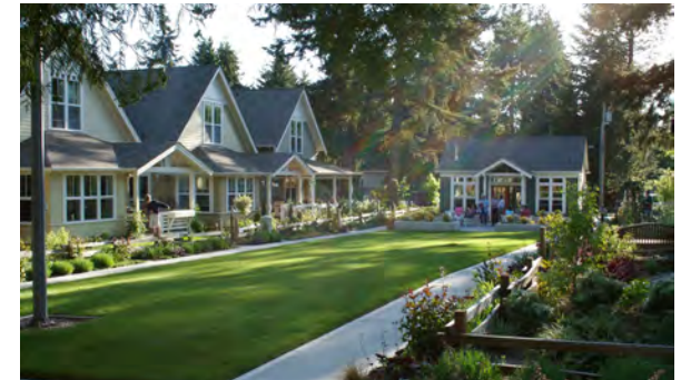
Single-family homes (Danielson Grove, Kirkland, WA)
