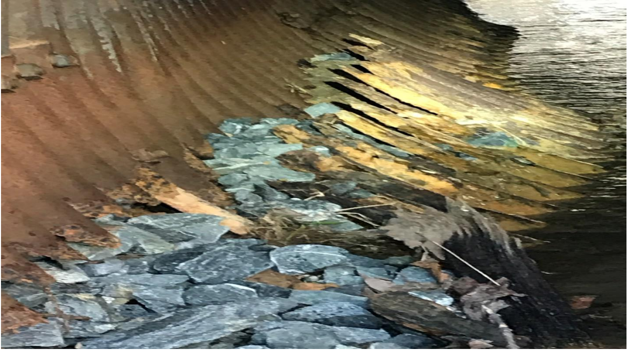
Stone placed in the voids to slow failure.
