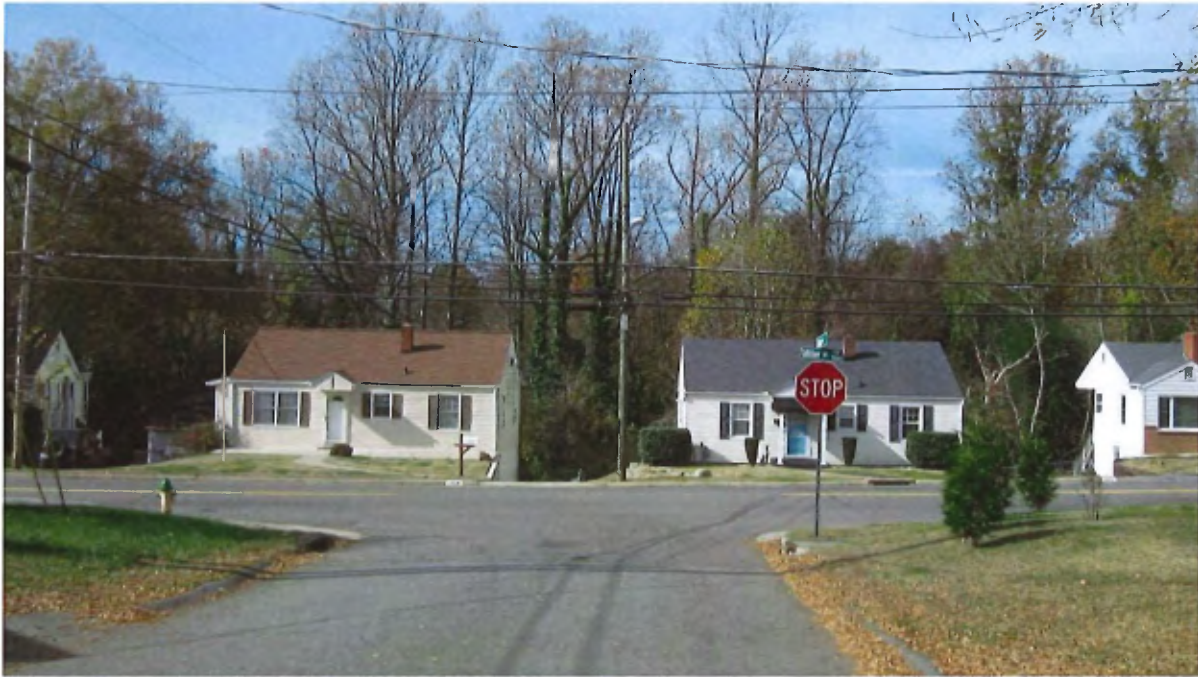
Dwelling on Miller Street from Boone Avenue
