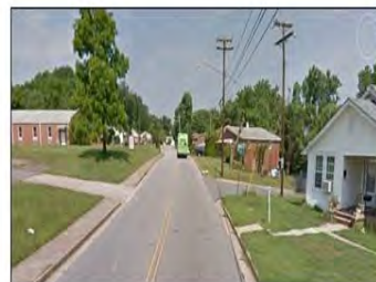
Douglass Street exits at a curve location on Dellabrook Road.
