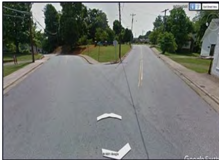
This “y” road configuration is a constant danger to drivers and pedestrians
