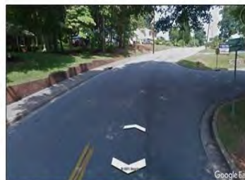
This entry point onto Emerald Street obstructs views of oncoming traffic.
