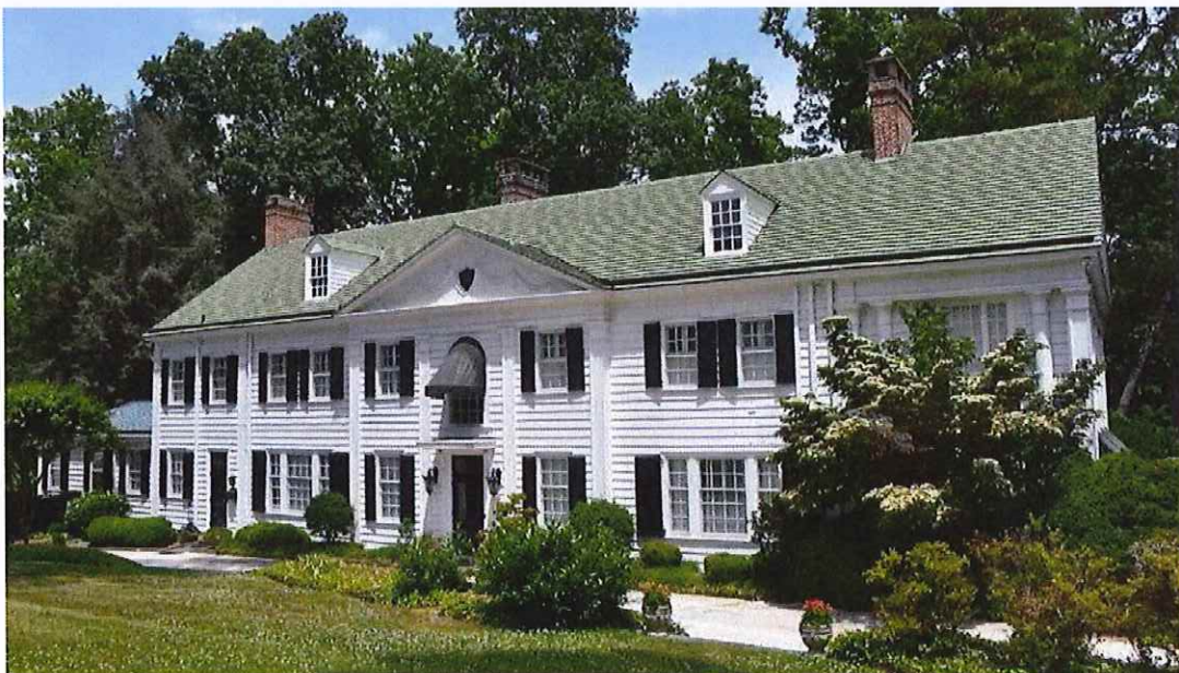
Façade (west elevation)
