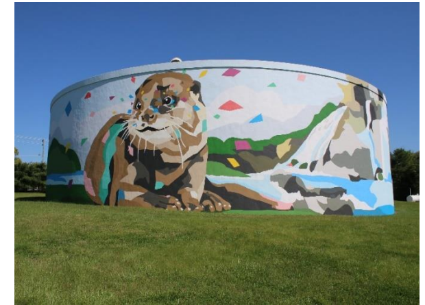
Sides Road Tank - 2015
