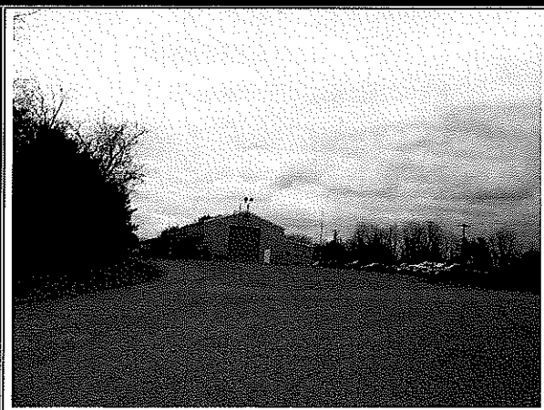
VIEW OF MAINTENANCE SHOP
