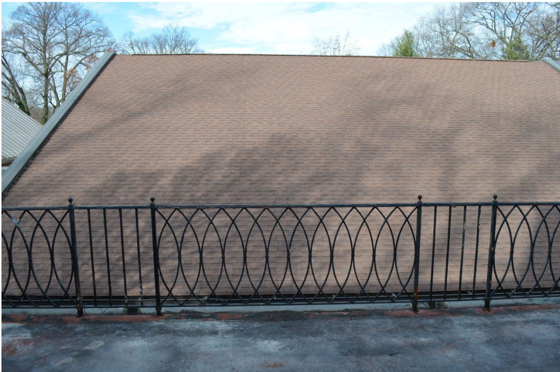
Rear Balcony Balustrade
