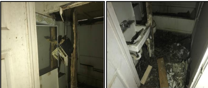
Internal photos were taken prior to No Trespassing signs placed. 12/24/2019
