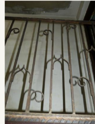
Rooftop stair detail of 301 W. 4 th
