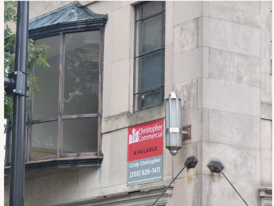
Exterior lighting and window detail
